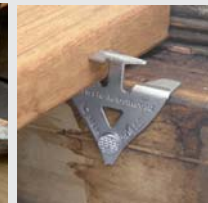
Nail the Sharktooth to the joist.
